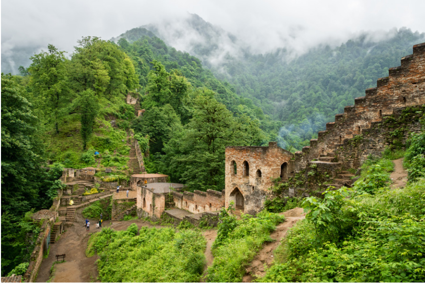
Figure 18.16 Rudkhan Castle, built by the Sassanids, rebuilt by the Nizaris (© Uskarp/Shutterstock)
